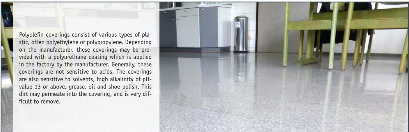
Polyolefin coverings consist of various types of plastic, often polyethylene or polypropylene. Depending on the manufacturer, these coverings may be provided with a polyurethane coating which is applied in the factory by the manufacturer. Generally, these coverings are not sensitive to acids. The coverings are also sensitive to solvents, high alkalinity of pH-value 13 or above, grease, oil and shoe polish. This dirt may permeate into the covering, and is very difficult to remove.
