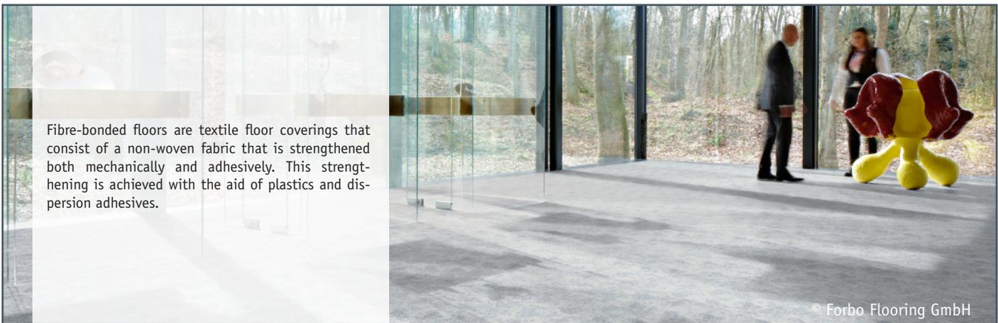
Fibre-bonded floors are textile floor coverings that consist of a non-woven fabric that is strengthened both mechanically and adhesively. This strengthening is achieved with the aid of plastics and dispersion adhesives.
