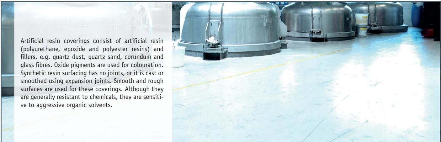
Artificial resin coverings consist of artificial resin (polyurethane, epoxide and polyester resins) and fillers, e.g. quartz dust, quartz sand, corundum and glass fibres. Oxide pigments are used for colouration. Synthetic resin surfacing has no joints, or it is cast or smoothed using expansion joints. Smooth and rough surfaces are used for these coverings. Although they are generally resistant to chemicals, they are sensitive to aggressive organic solvents.
